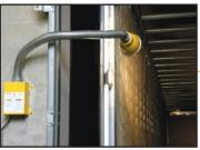
Interior dock lights can be powered through control panel and can be programmed to operate before dock operations begin.
