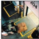
Leveler functions are interlocked with other dock devices to prevent operation until all the safety systems are operational and the dock doors are opened.
